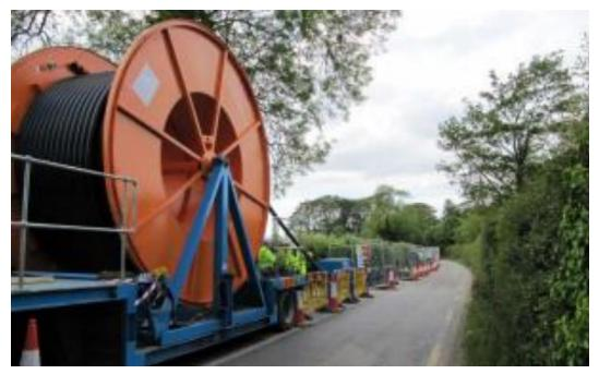
Figure 4.13: Cable Drum at Joint-bay location
